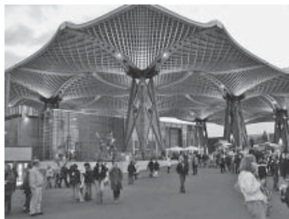
Figure 9 Modern timber construction Expo Roof - Hannover exhibition grounds
